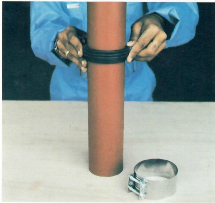
Step 4 – Fit other pipe or fitting into rubber seal
