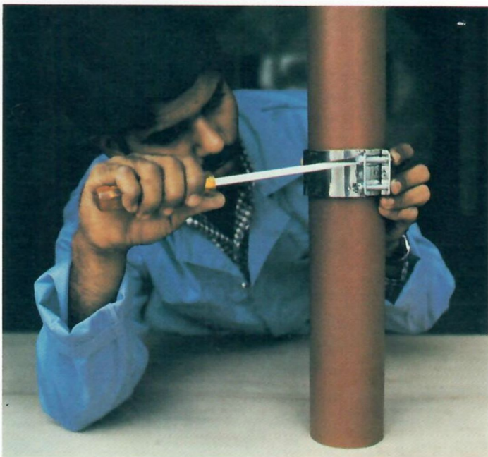
Step 6 – Tighten steel fastener securely
