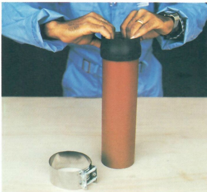
Step 2 – Fit rubber seal to end of pipe for fitting
