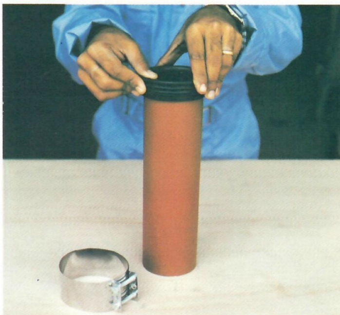
Step 3 – Roll back free end of rubber seal
